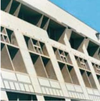
Natural stone cladding with large and varying cavities can be attached without problems, using the LUTZ sub-structure systems.
